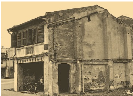
Figure 3: Before demolition in 1974
